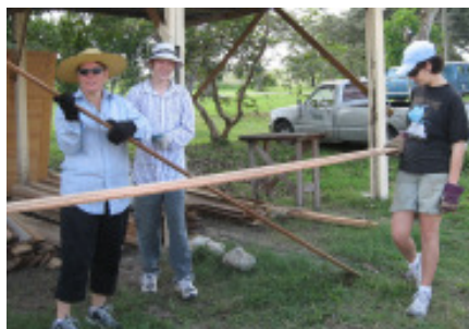
Measuring out the siding for the walls.
