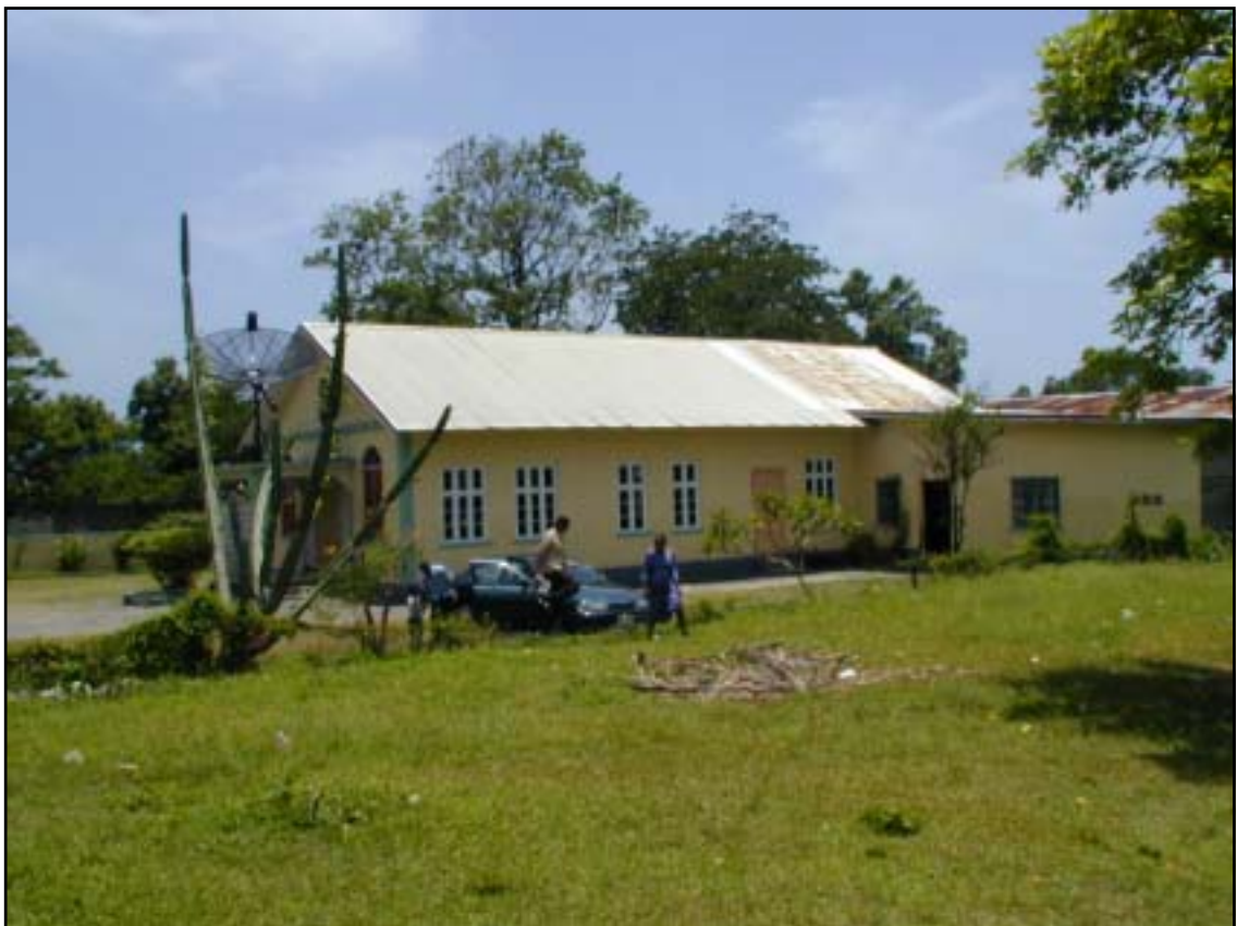
The Buff Bay Church and EEC site
